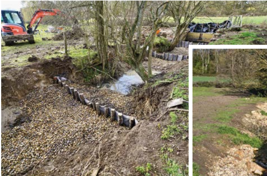
The Shalbourne fish pass during and after construction. Credits: Rupert Kelton ARK and Cain Bio Engineering
