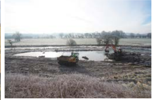
Constructing the wetland at Fyfield, January 2023. Credit: Rupert Kelton ARK
