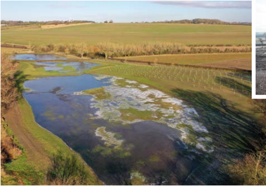
Aerial View of the new Wilton wetland, January 2023. Credit: Cain Bio Engineering
