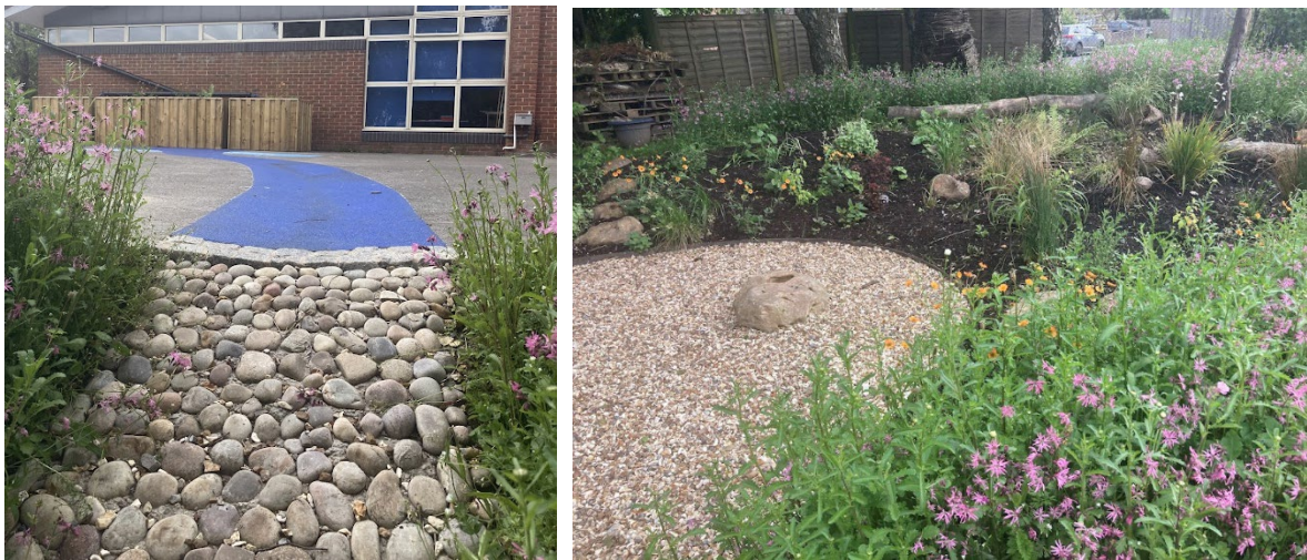
Great Bedwyn School Rain Garden takes rain from the roof, through rain planters, across the playground and into a planted rain garden.
