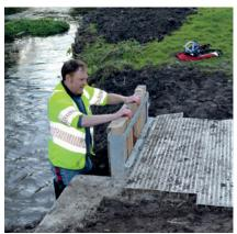
Before Christmas we completed the long-awaited fish pass at Stitchcombe Mill. Working in partnership the Environment Agency and the River Keeper, and using local contractors, we have built a new channel which allows fish to bypass the sluices that feed into the weir pool. The new pass will mean that fish can swim up and down the river whatever the state of flow, avoiding the obstacle that the sluice structure creates for them.
