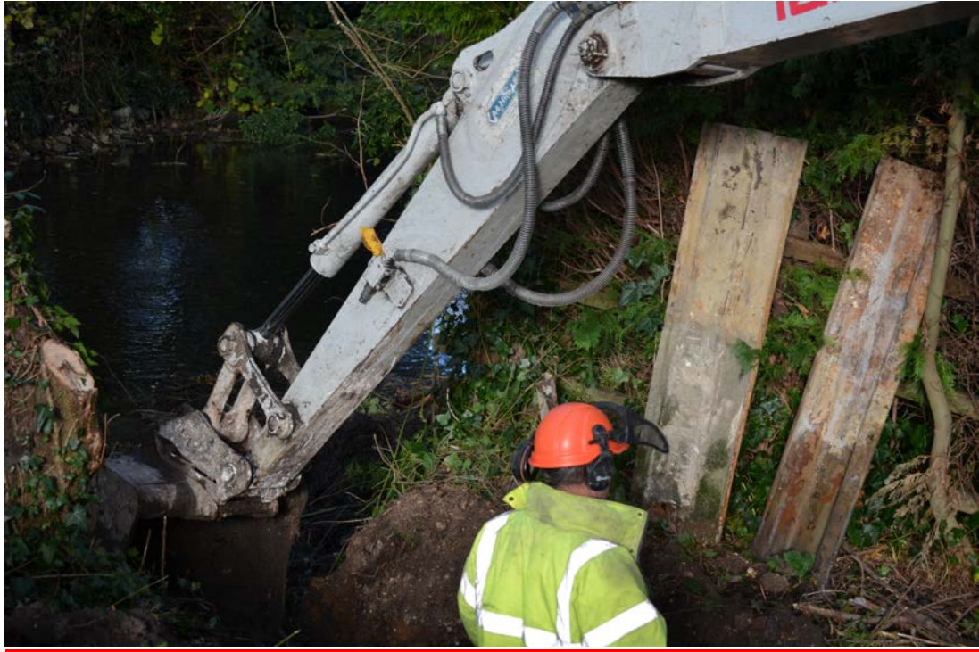
Excavating the new channel for the fish pass
