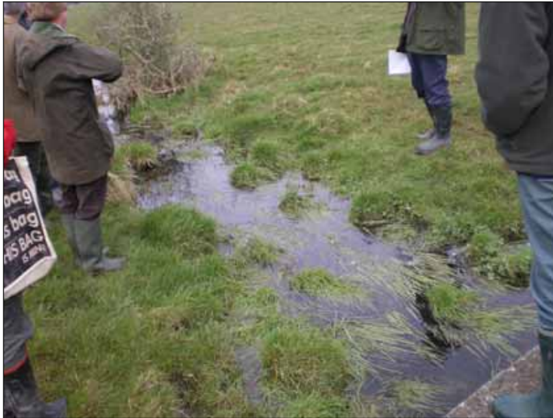
Bridge in bottom right corner of picture is constructed over a winterbourne spring which may only flow for a few months.
