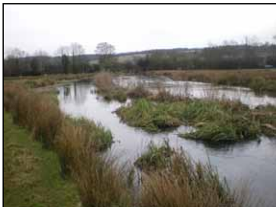
Kennet at Hoppers Lane, showing Berm and backwater, constructed in 2002 as part of the Upper Kennet Rehabilitation Project.
