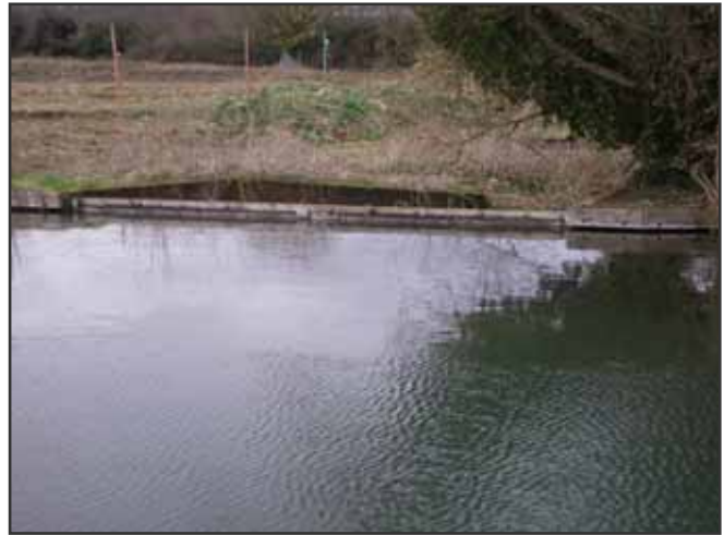
Boards across a spillway leading directly to River Dun. Boards are inserted or removed by British Waterway staff to control the canal level.
