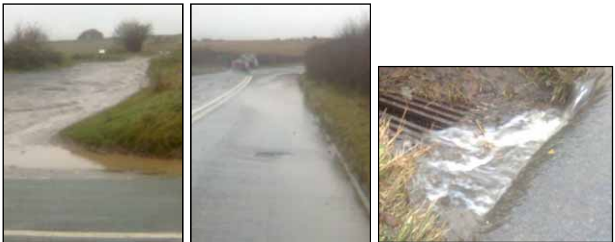
Heavy rainstorm causing sediment-laden runoff to stream from the Ridgeway, onto the A4 and down the drain to the Kennet (2008). Farmers feel that they are blamed for this runoff.
