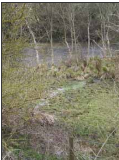
Photo: Leak from canal (at bottom of picture, out of shot) to River Dun (at top of picture).
